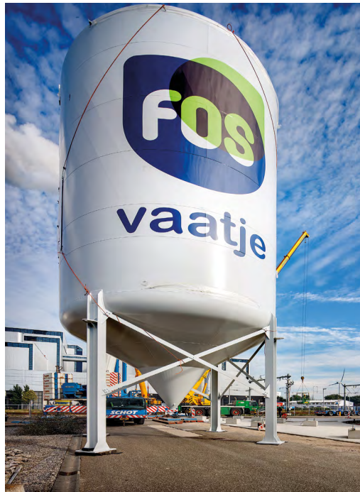
FosVaatje silo containing struvite.
